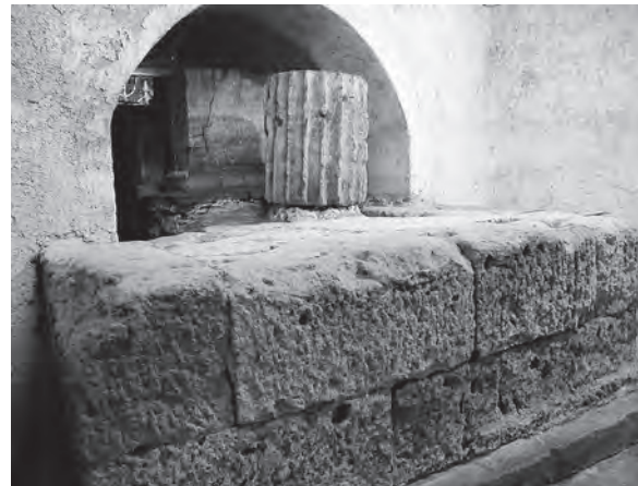
FIG. 3. The current state of the monument in the basement of Via San Martino ai Monti 8. The column drum on top of the podium is not in situ and was placed on top of the podium at some point after its excavation from the surrounding area.
