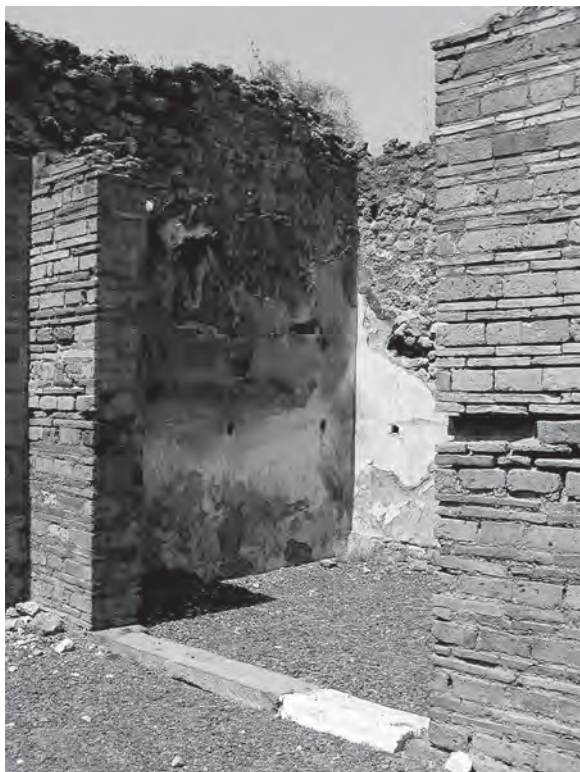
FIG. 8. House VI.13.13, Pompeii, view of the right ala , which is closed off by jambs in opus vittatum mixtum and a door with a threshold. Note the holes for shelving along the side and back walls.
