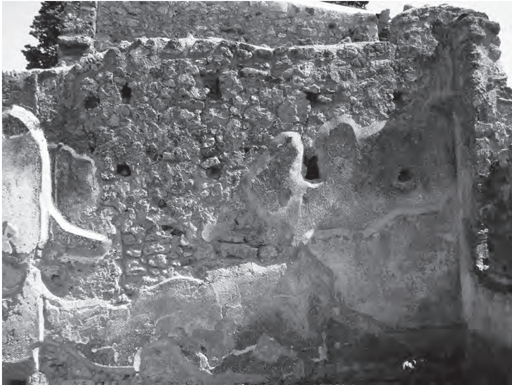
FIG. 11. Casa del Labirinto (VI.11.10), Pompeii, left ala on the Corinthian atrium, detail of south wall with holes for shelves.
