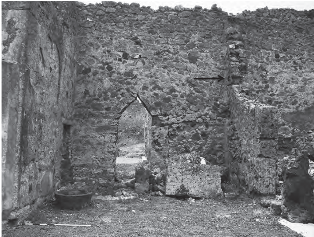
FIG. 18. Casa del Forno di Ferro (VI.13.6), Pompeii, left ala with door communicating with House VI.13.2, including the base of the staircase; the hole for the loft in the north wall is indicated with an arrow.
