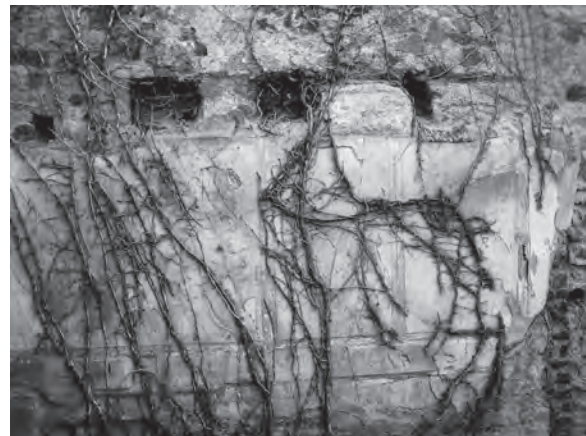
FIG. 14. Casa di Pupius Rufus (VI.15.5), Pompeii, detail of sockets for loft in north wall of left ala ; horizontal groove left by wooden planks is visible.
