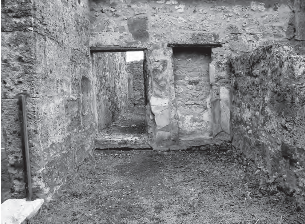
FIG. 9. Casa del Chirurgo (VI.1.10), Pompeii, right ala with door and niche in the south wall.
