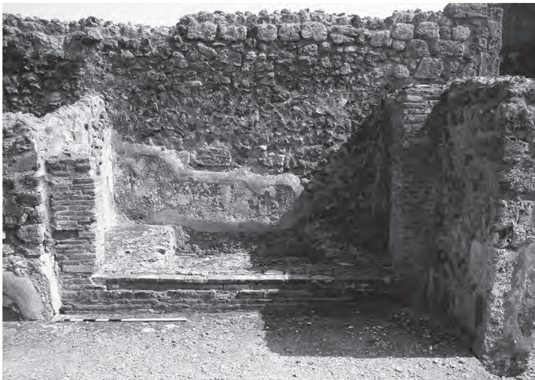
FIG. 5. Casa di Adone Ferito (VI.7.18), Pompeii, view of the ala with masonry base and brick jambs.
