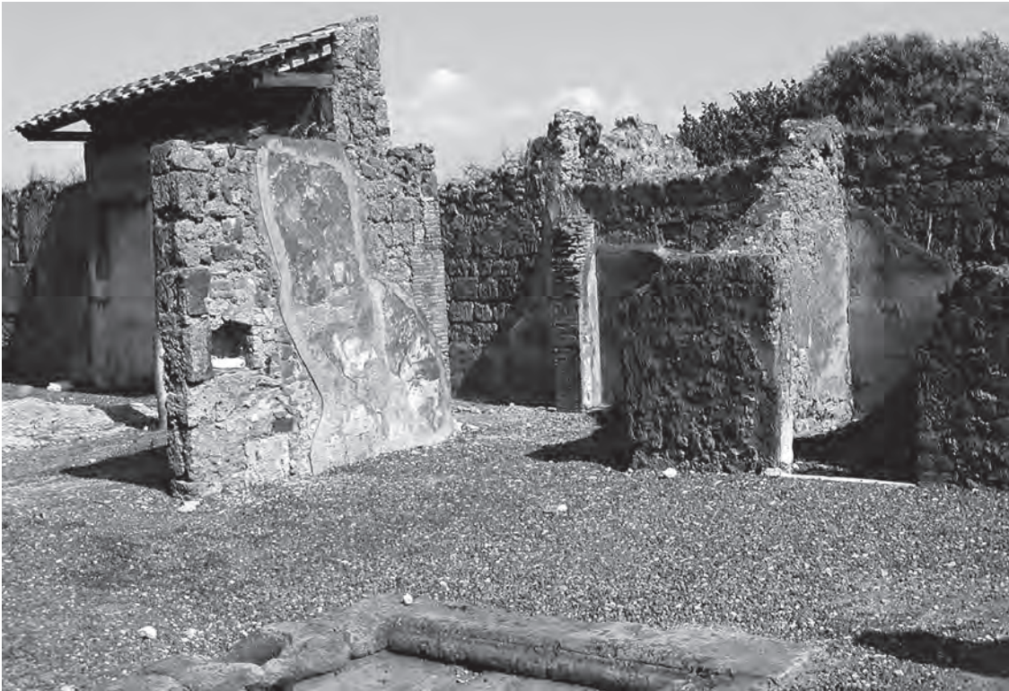
FIG. 21. Casa del Granduca Michele (VI.5.5), Pompeii, view of the alae across the atrium with large opening in the east wall; the jambs are reinforced in opus latericium .
