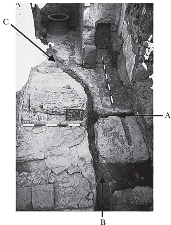
Fig. 5. The water-pipe trenches and location of the junction box in the praefurnium: a , aqueduct water enters the house; b , water pipe leading to the fountains in the Narciso atrium (27), small peristyle (14), and the Consolare atrium (2); c , water pipe leading to the swimming pool in the large peristyle (39)
