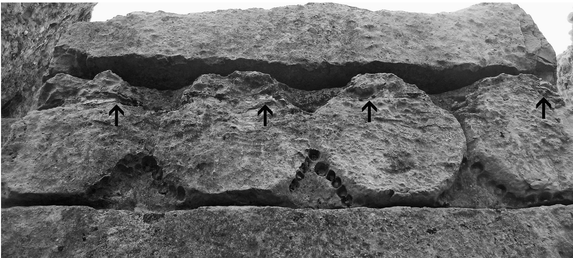
Fig. 1. Detail of the entablature of the Lion Gate relief, showing the location of tubular drill holes and saw marks. The arrows indicate the erroneous saw cut and the unknown filling material within it.
