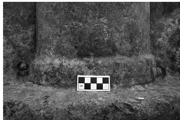
Fig. 3. Detail of the base of the column, showing drill holes.
