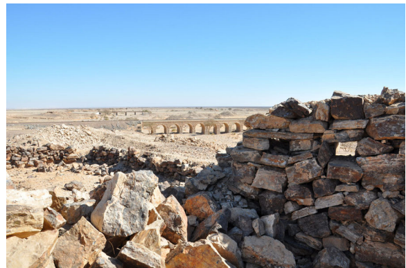
Fig. 79. Makin's Fort, an outpost that once protected the Hijaz railway line; view of loopholed wall across wadi to multispan bridge carrying the railway (© N. Saunders; The Great Arab Revolt Project).
