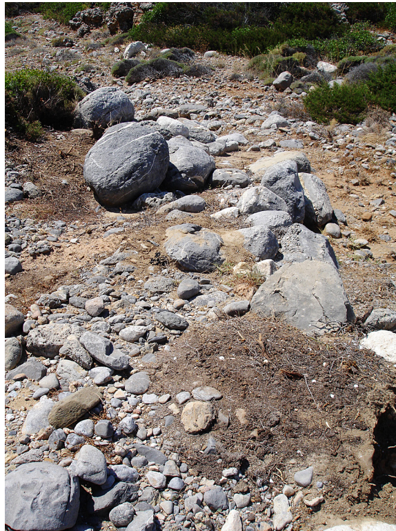
Fig. 6. View to west of inner dam.
