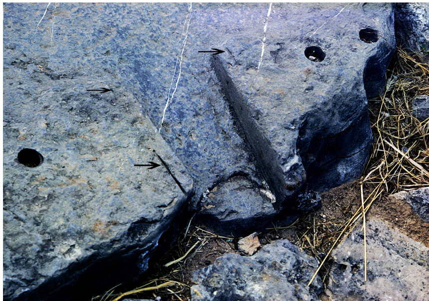
Fig. 5. Exit channel for water in northeastern corner of bathing slab at Tiryns. Note preliminary saw marks at arrows.
