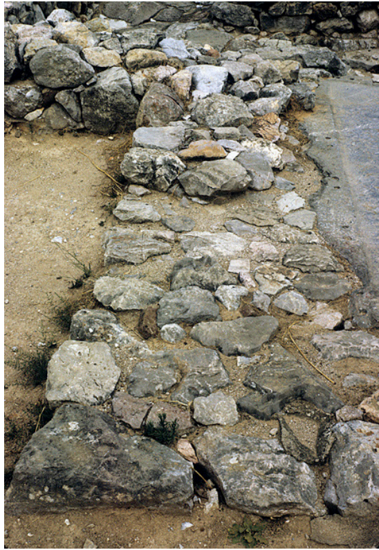
Fig. 4. Denuded north wall looking east (terracotta containers are missing in this 1974 photograph).
