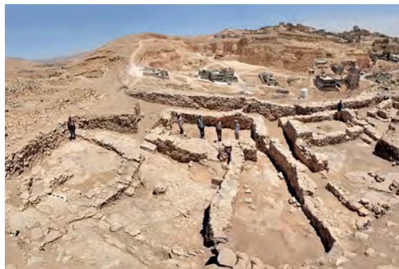
Fig. 9. General view (from the south) of the Early Bronze (EB) III B Palace B at Khirbat al-Batrawy. The palace was erected inside the EB II–III main inner-city wall (courtesy Khirbat al-Batrawy Excavations).
