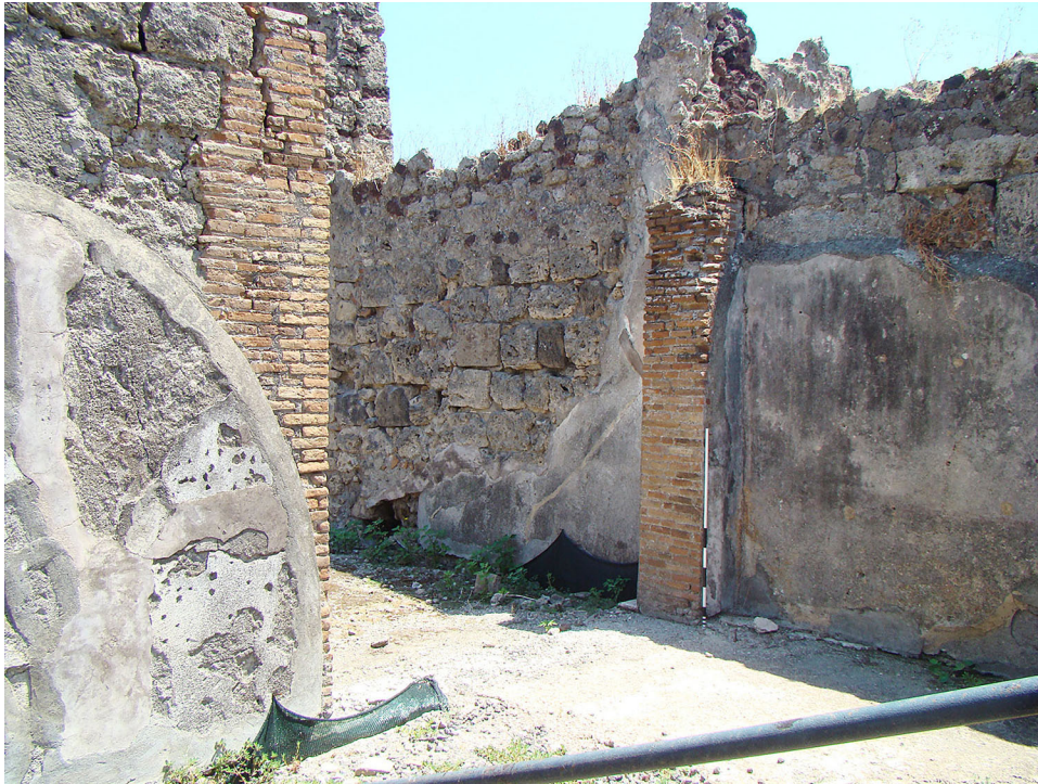
Fig. 10. Casa del Granduca Michele (VI.5.5), Pompeii, opening in east wall of ala with jamb reinforcements in opus latericium .
