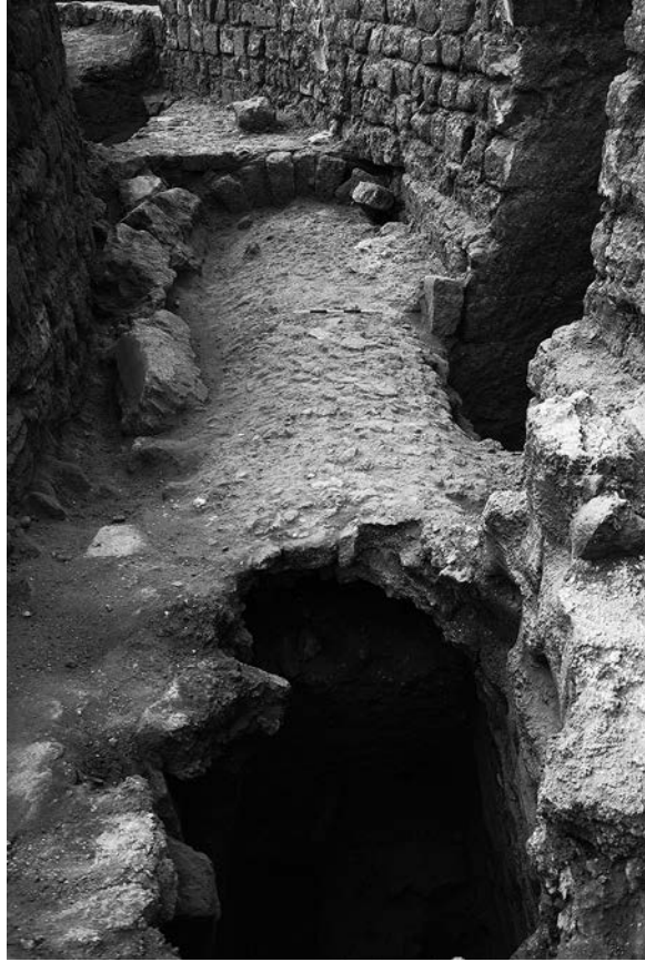
FIG. 13. The sewer running below the rear wall of the Severan (phase 5) bouleuterion/odeum (view to the southeast).
