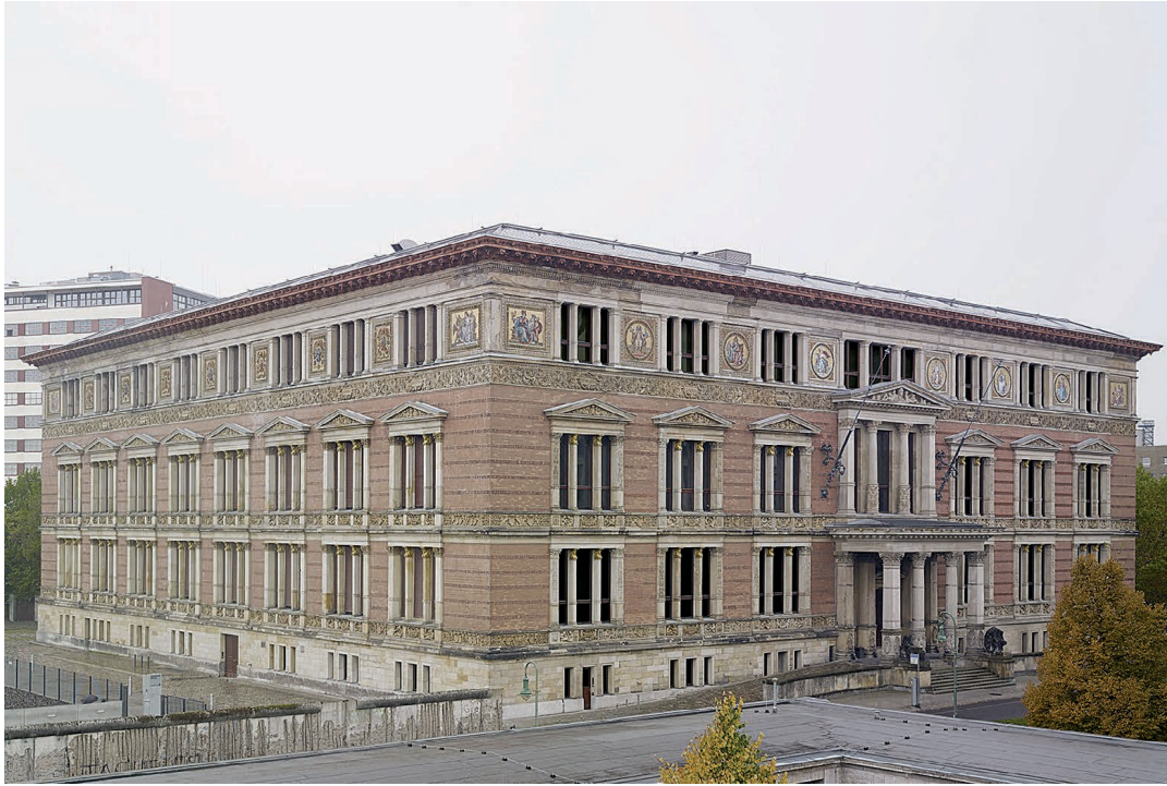
FIG. 1. Gropius Bau, Berlin. On the street in front of the building are remains of the former Berlin Wall, and behind it are excavated remains of the headquarters of the Secret State Police (Gestapo), part of the open-air exhibition Topography of Terror (C. Ruggaber; © Berliner Festspiele).
