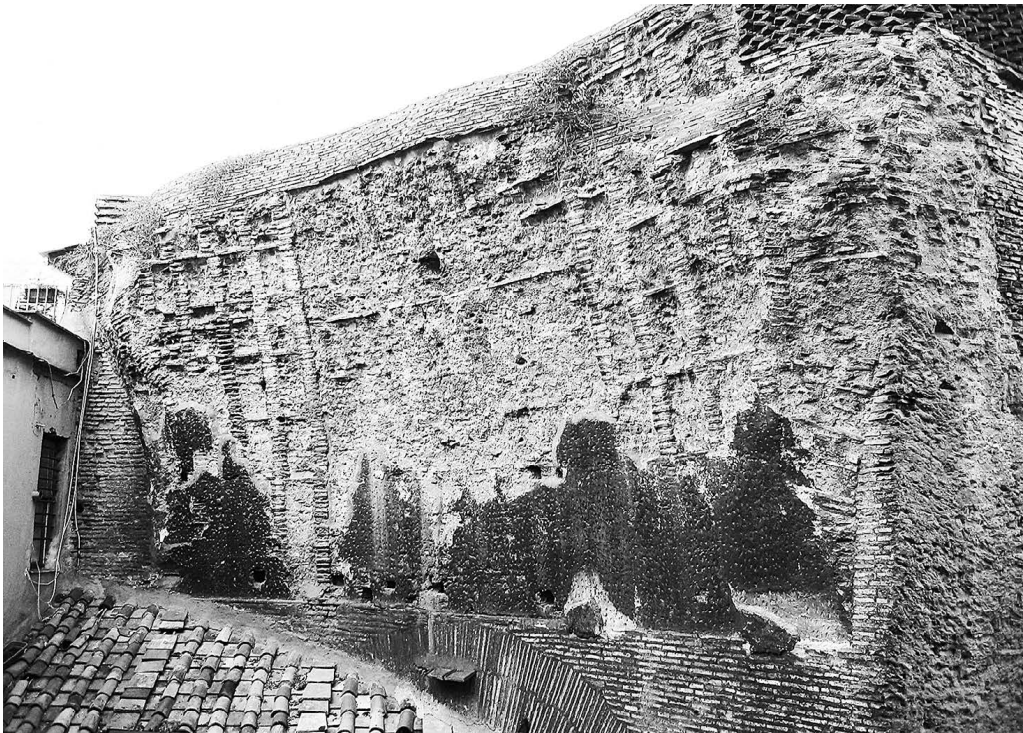
FIG. 9. Remains of the central dome of the Thermae Agrippae, the so-called Arco della Ciambella, showing a pattern of fourth-century C.E. lattice ribbing (courtesy L. Lancaster).
