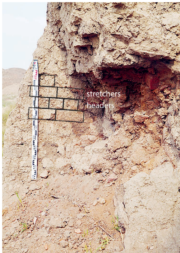
FIG. 13. Exterior wall of the L14 structure with bricks laid in the English bond pattern, looking west.
