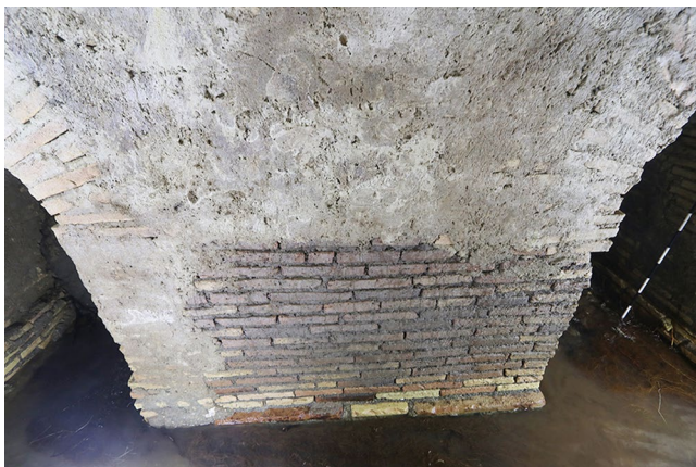
FIG. 8. East face of Pier 11. Most of the bricks below arch level appear to be ancient (R.B. Gorham).
