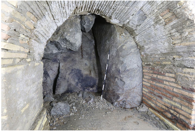
FIG. 4. Arch 8, looking west. Most of the piers and arches are positioned snugly against the rock face (R.B. Gorham).
