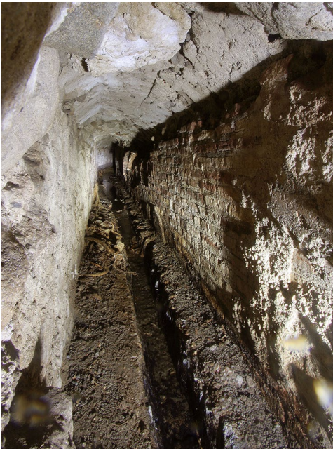
FIG. 12. South feeder channel looking south (R. Taylor).
