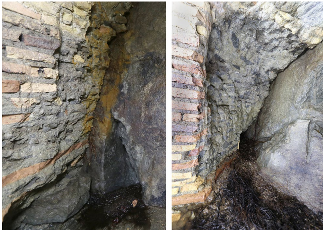
FIG. 5. Hacked concrete cores: left , behind Pier 5; right , behind Pier 11. Tiers of aggregate and visible bipedales running through the thickness of the piers demonstrate that the cores are Roman (R.B. Gorham).
