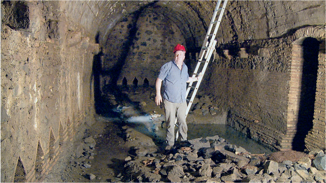
FIG. 15. Botte Micciario along the Fosso Boccalupo; part of the 17th-century Acqua Paola. Springwater emerges from the peaked openings low in the wall on three sides (M. O'Neill).
