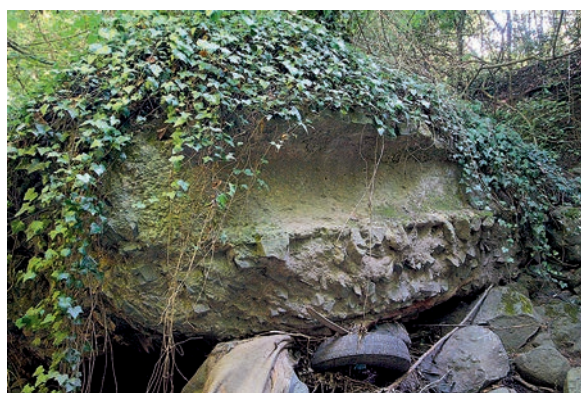
FIG. 23. A fallen segment of the water channel from the first bridge above Passo del Guardiano as seen in 2011 (R. Taylor).
