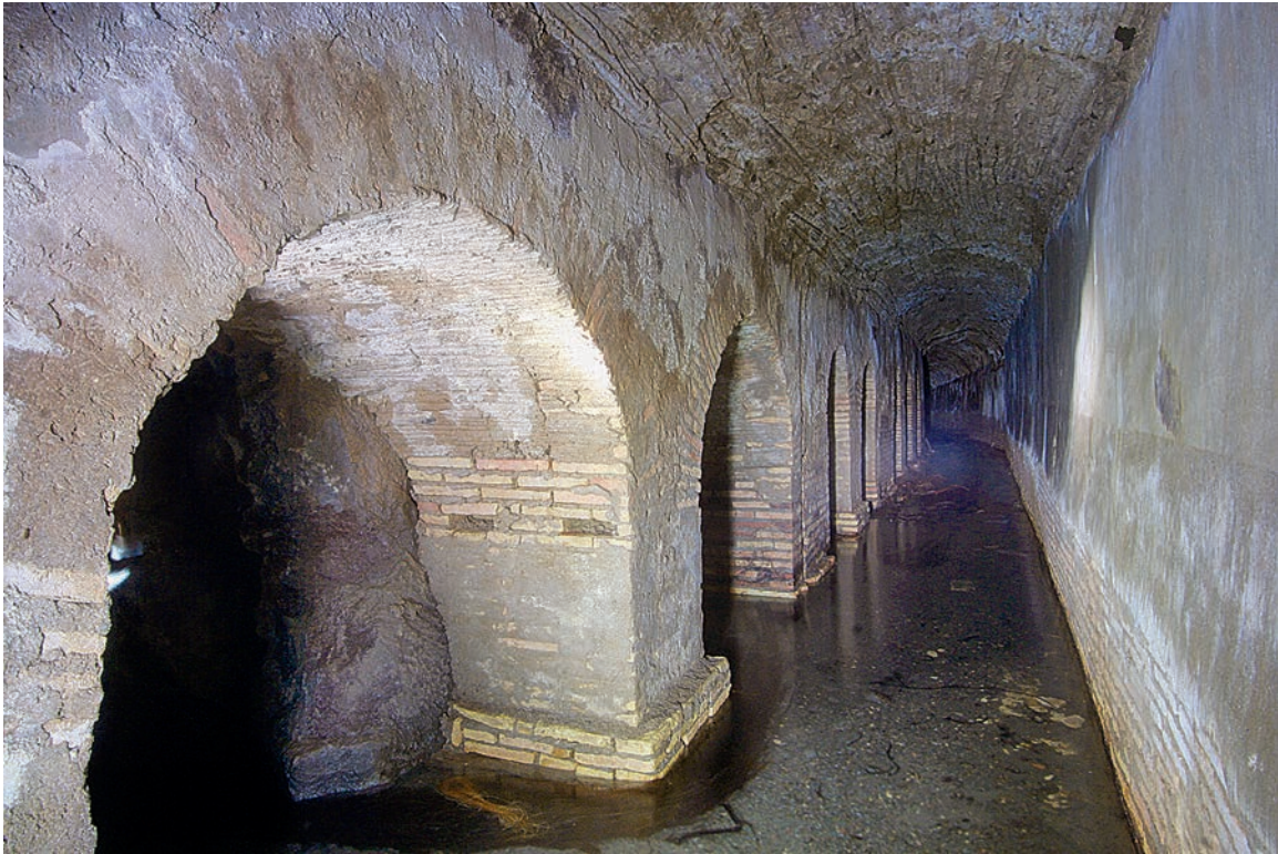
FIG. 12. Main gallery of the long springhouse, looking north (R. Taylor).
