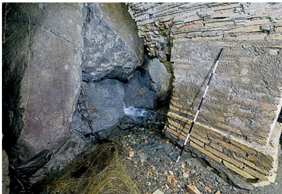
FIG. 13. Water emerging from behind Pier 4 in the main gallery at Vicarello, looking northwest (R.B. Gorham).
