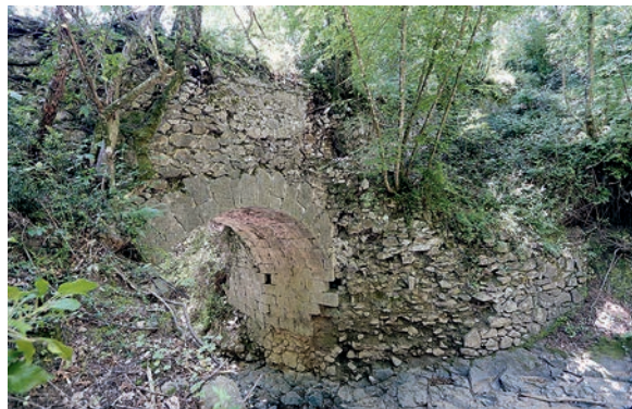
FIG. 22. The second, later bridge over the Fosso della Calandrina at Passo del Guardiano, looking southwest (R. Taylor).
