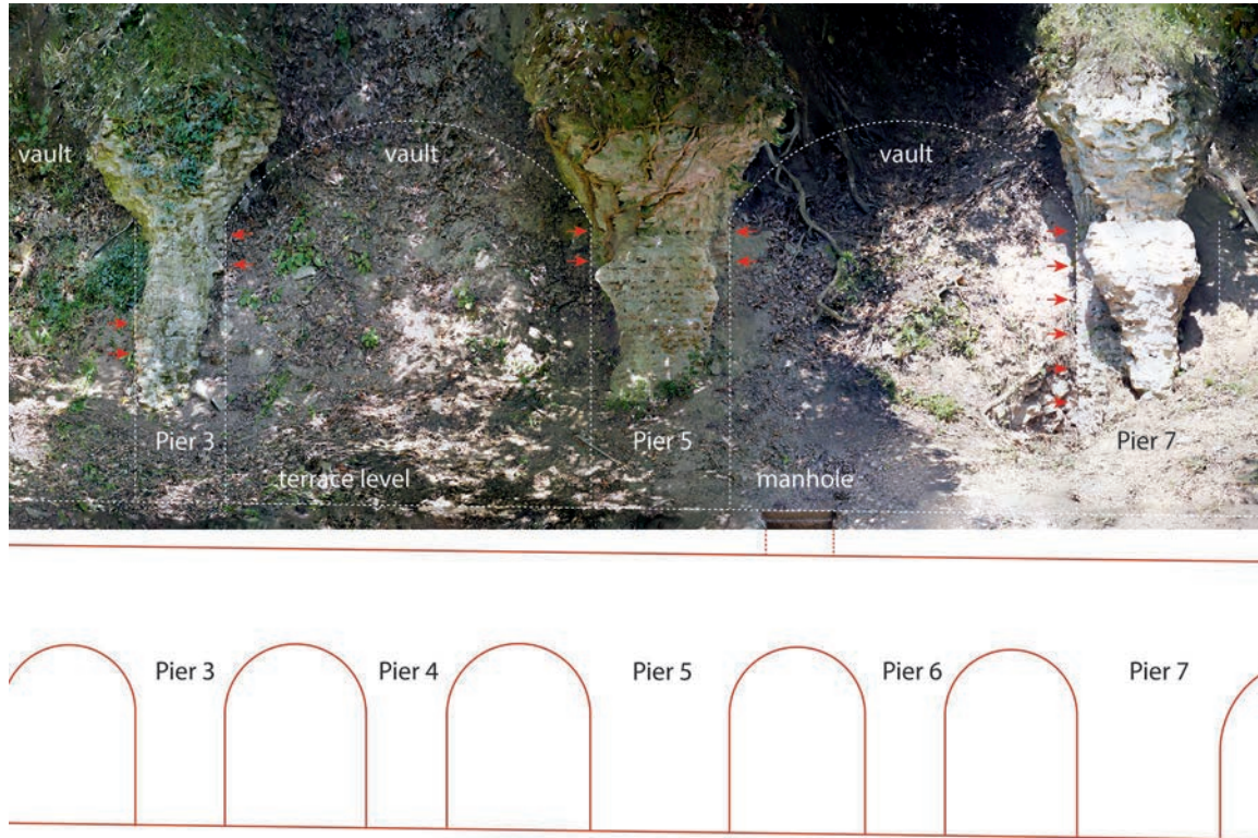
FIG. 9. Elevation view of the multivaulted structure aligned with a section drawing of the subterranean main gallery of the long springhouse. Piers 3, 5, and 7 appear to continue from the floor of the subterranean main gallery up through the vaulted structure. Red arrows indicate visible brick faces (photogrammetric models by R.B. Gorham; composite by R. Taylor).
